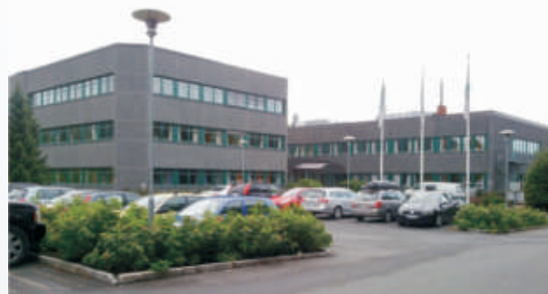
Comex Headquarters located in Norway
